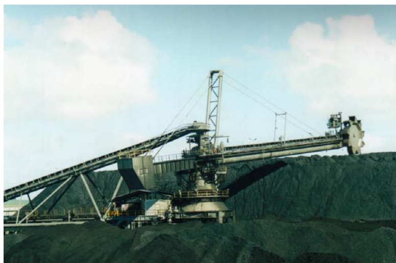
Figure 5 - 4000tph Stacker Reclaimer
